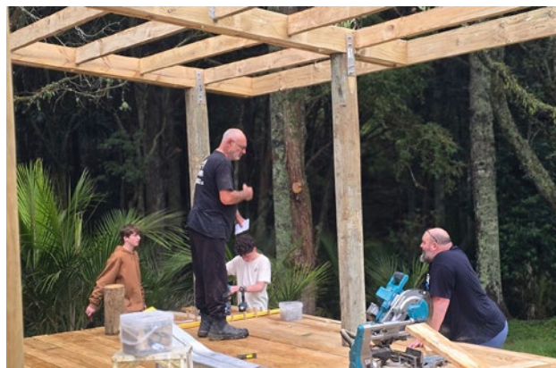
The Brains Trust – Front left is Grant Dobbyn [Dobbyn Builders owner] front right is Koen McGee [BBMK Builders owner].
